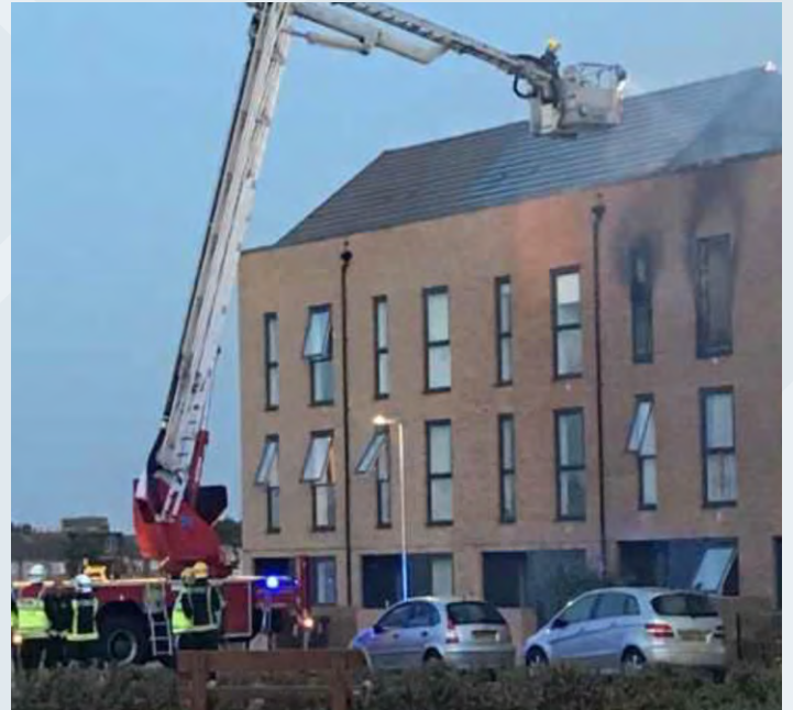
2 Presence of solar panels identified
