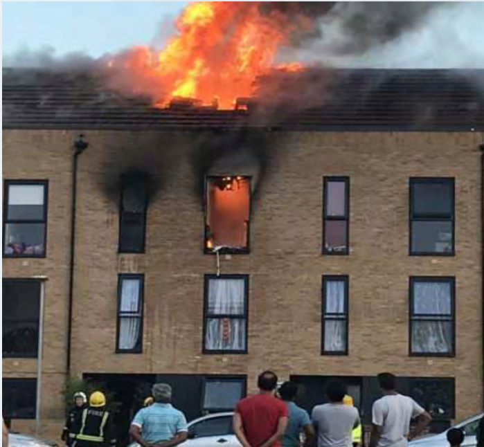
1 Mid terrace house fire
