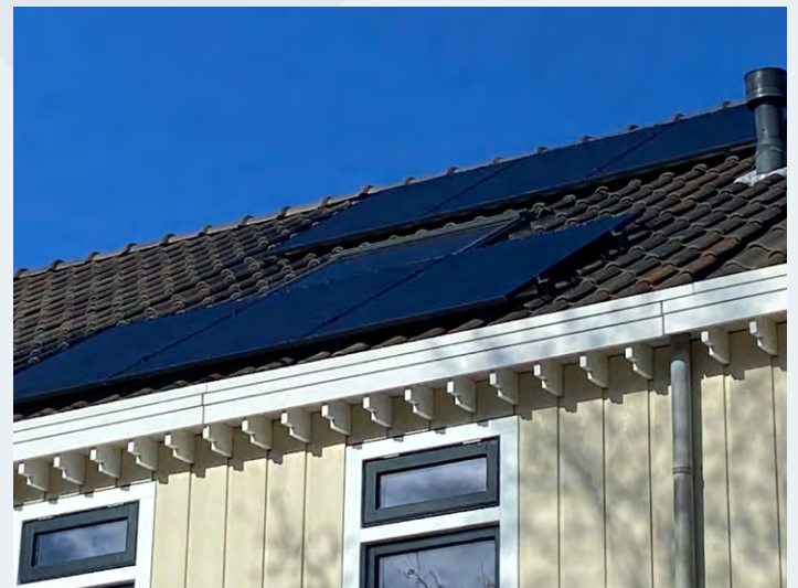
5 PV System safely de-energised
